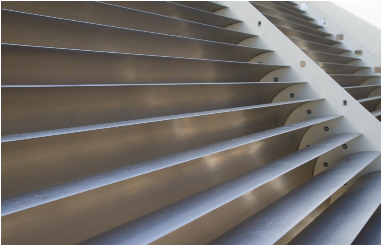
Fig. A.1.4 The illustration showcasing the method of attaching the vanes (TTE-TV) to the diagonal metal plates – the diagonal supports of the turning section (TTE-TSCDS and TTE-TSSDS).
