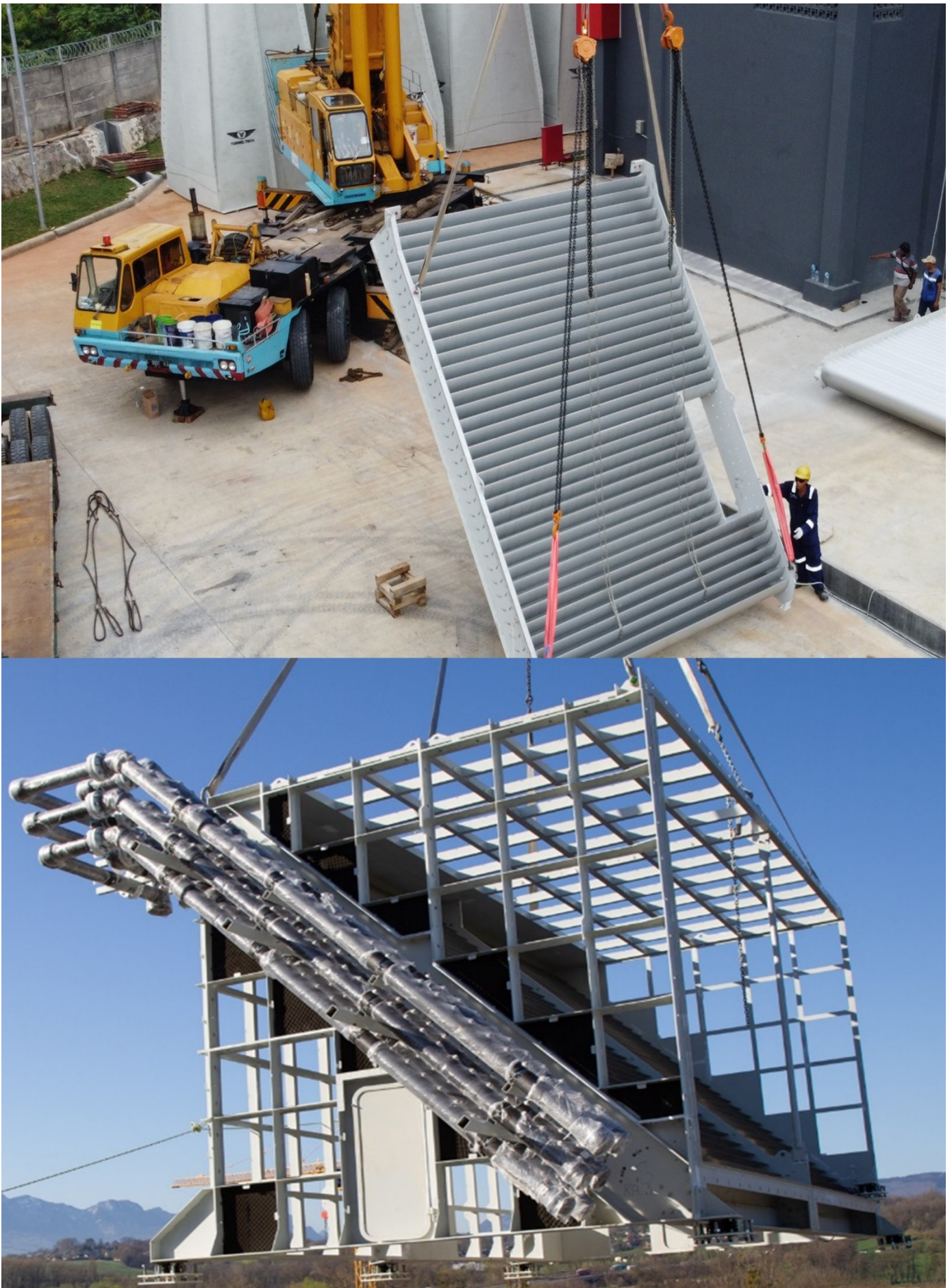
Fig. 2.12 Turning section doors: top - vane door,. bottom – maintenance door.
